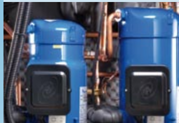
Higher efficiency and quieter operation thanks to scroll compressors
